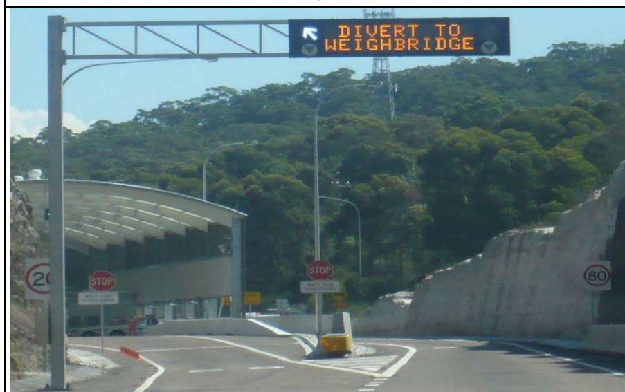
Exhibit 8: The screening lane at Mt White southbound heavy vehicle checking station
