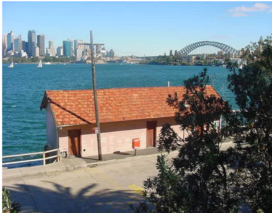
Cremorne Tram Shed
